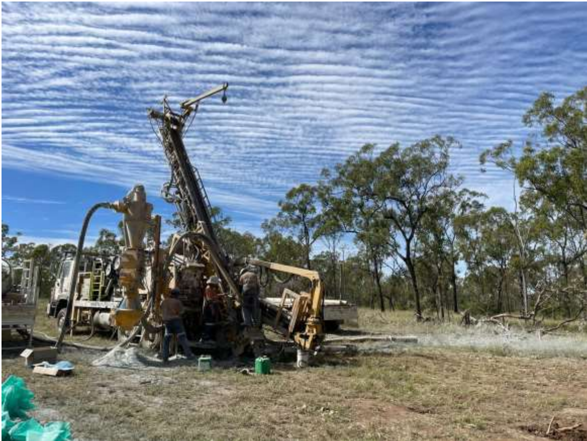
Figure 2: Drill Rig in Queensland
