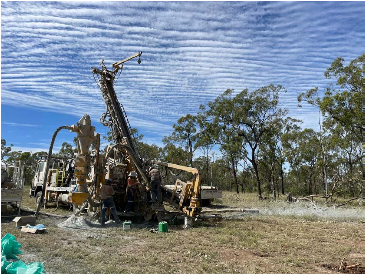
Figure 2: Drill Rig in Queensland
