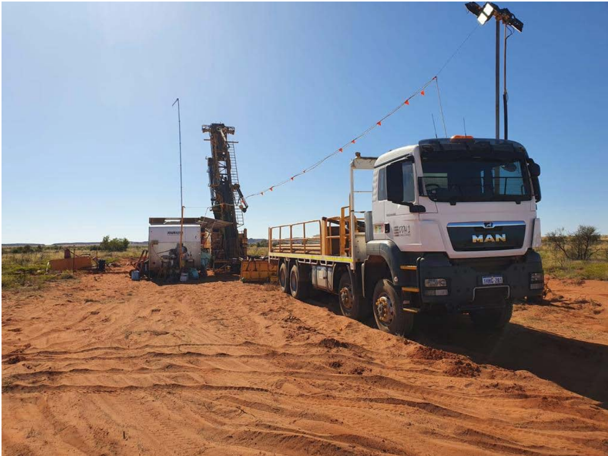
Figure 1: Drilling at Red Setter
